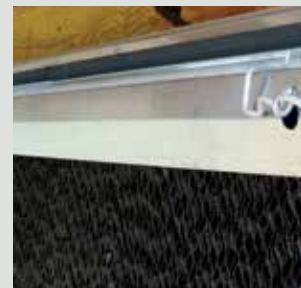
The spray bar bracket and water deflector insure pads are uniformly wet.
