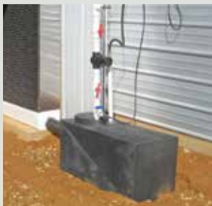
A roto-molded holding tank offers increased water storage capacity.
